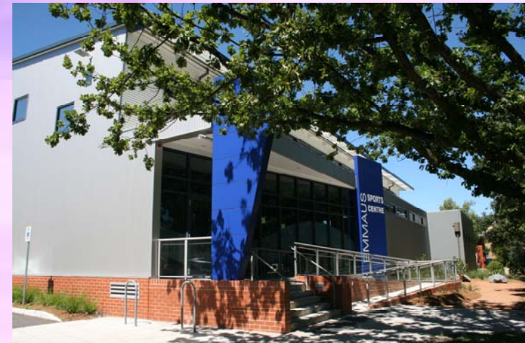
Gymnasium completed and in use.
